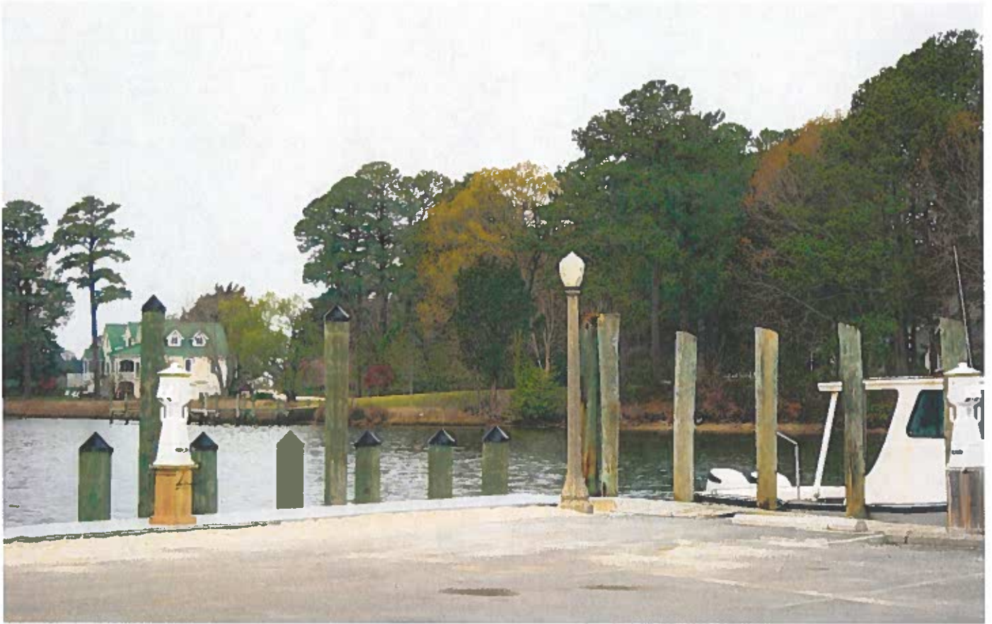
The existing wharf
