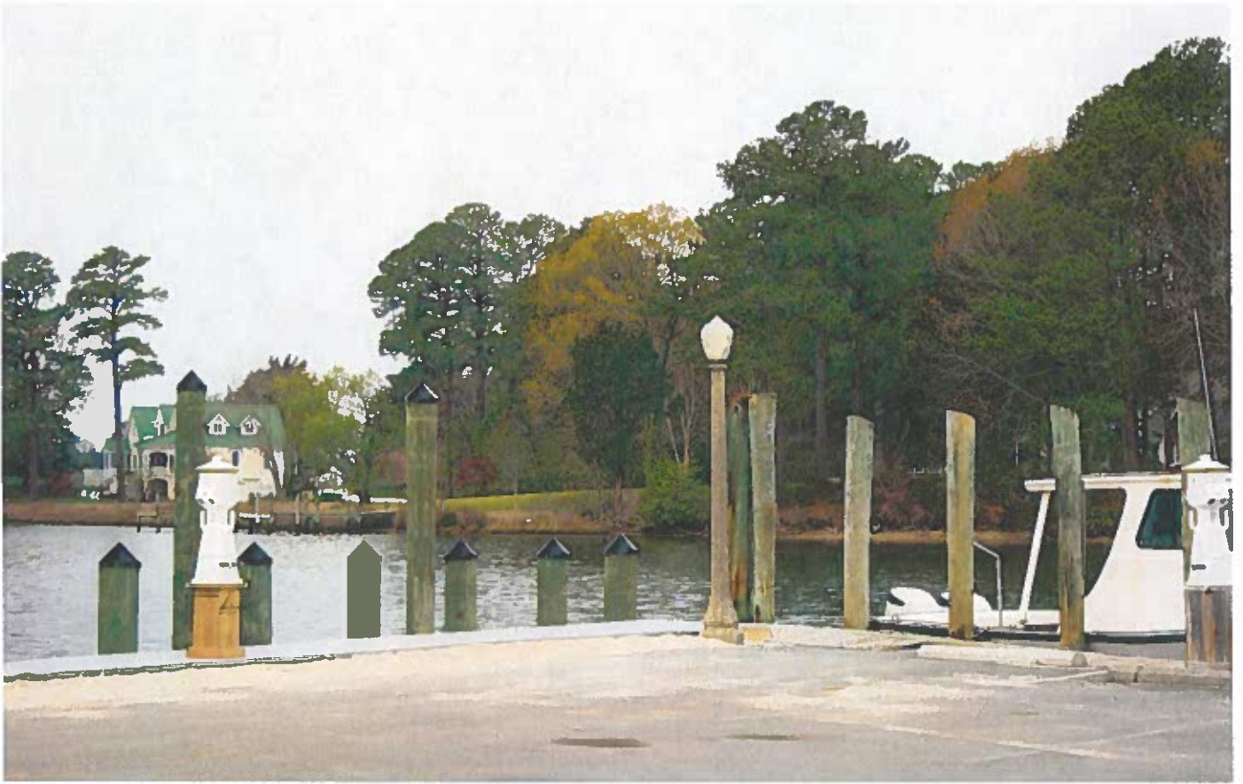
The existing wharf
